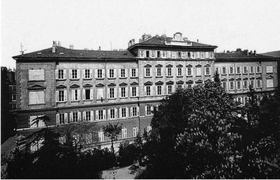
The building of the I.R. Accademia di Commercio e Nautica of Trieste at the beginning of the 20th century
