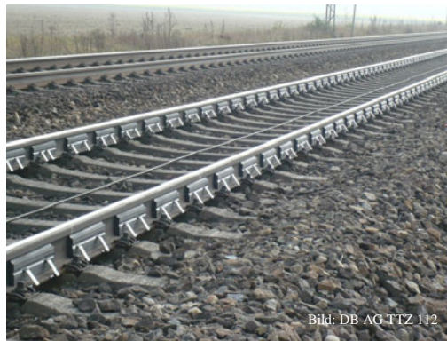
Fig. 4. Rail dampers are mounted on an existing track near Augsburg (color figure online)
