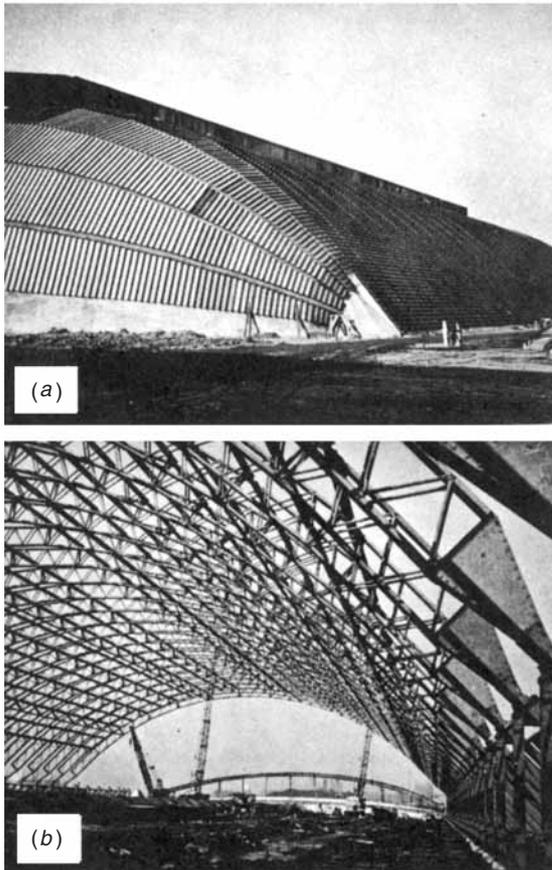
**Figure 1.9** Hangar-type arch structures using cold-formed steel sections. (Courtesy of Armco Steel Corporation.)<sup>1,6</sup>
