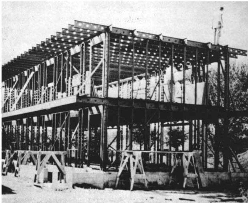
**Figure 1.3** Building composed entirely of cold-formed steel sections. (Courtesy of Penn Metal Company.)<sup>1,7</sup>
