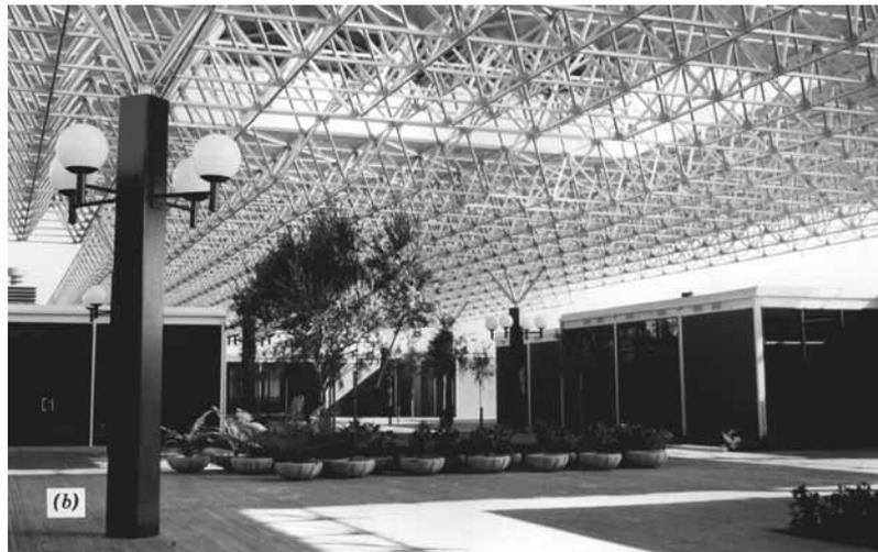
**Figure 1.6** Cold-formed steel sections used in space frames. (Courtesy of Unistrut Corporation.)
