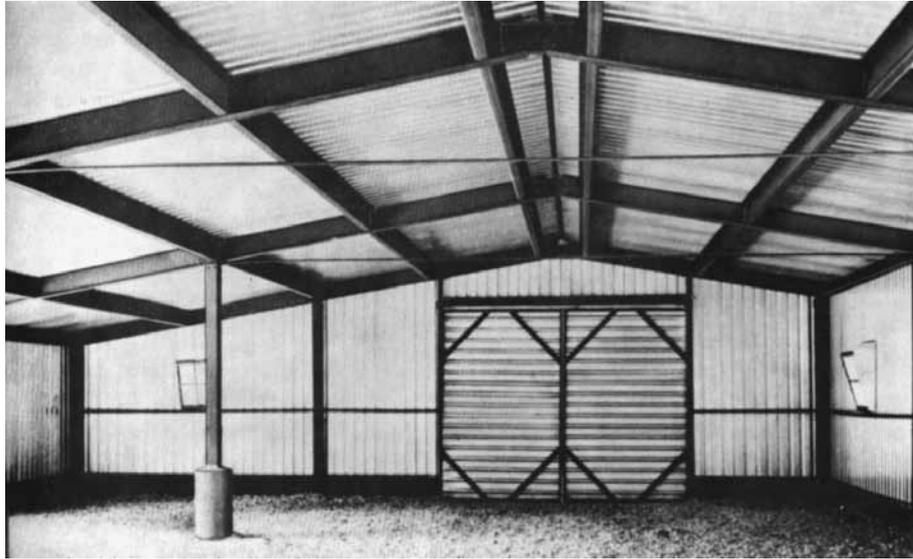
**Figure 1.20** Small building made entirely of cold-formed sections. (Courtesy of Stran-Steel Corporation.)<sup>1,6</sup>
