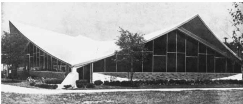
**Figure 1.14** Hyperbolic paraboloid roof of welded laminated steel deck. (Reprinted from *Architectural Record*, March 1962. Copyright by McGraw-Hill Book Co., Inc.)<sup>1.79</sup>
