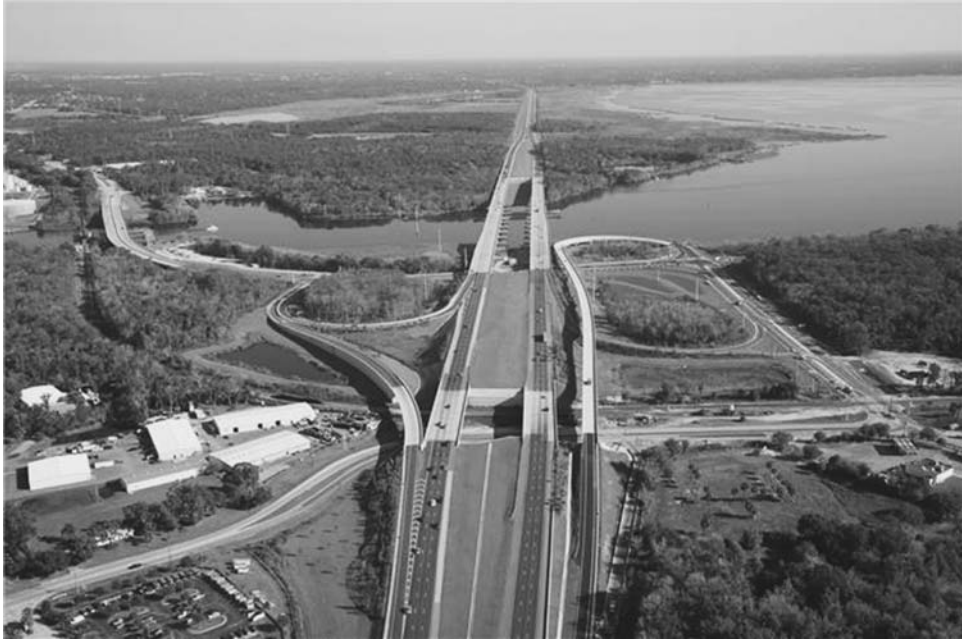
Interstate 4 and 17/92 intersection in Sanford, Florida
