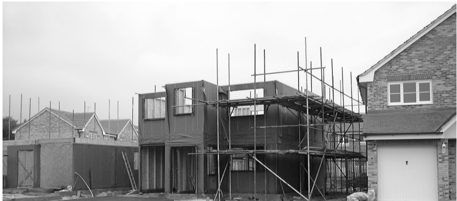
Photograph 1.1 Timber framed construction (courtesy of D. Johnston).
