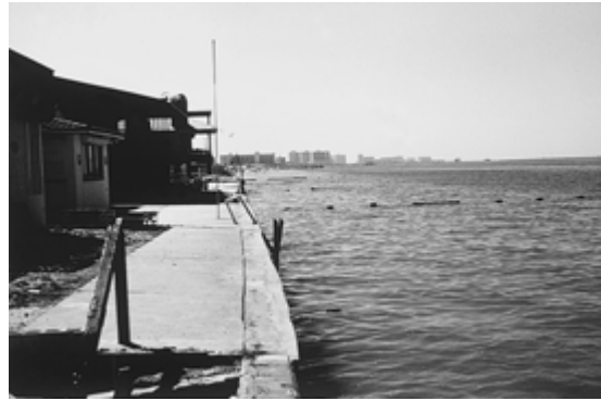
Fig. 1.10 Photograph of a seawall designed to protect the coast from erosion. These features are designed to stop erosion along the shoreline and to protect buildings or infrastructure that is close to the shoreline
