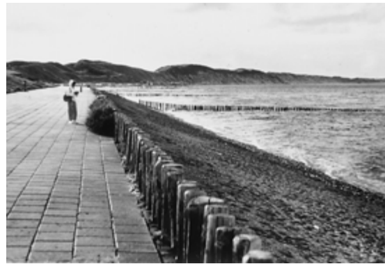
Fig. 1.11 Photograph of a dike along the Netherlands coast on the North Sea. Such structures protect the adjacent land, which is below sea level, from flooding. Like many of the dikes, this one supports a roadway. Some are used to graze sheep and cattle.
