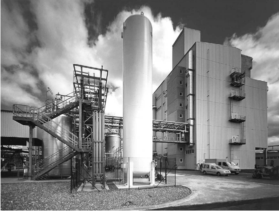
Figure 1.2 Strobilurin plant for BASF Schwarzheide GmbH with an order value of 14.9 million €.
