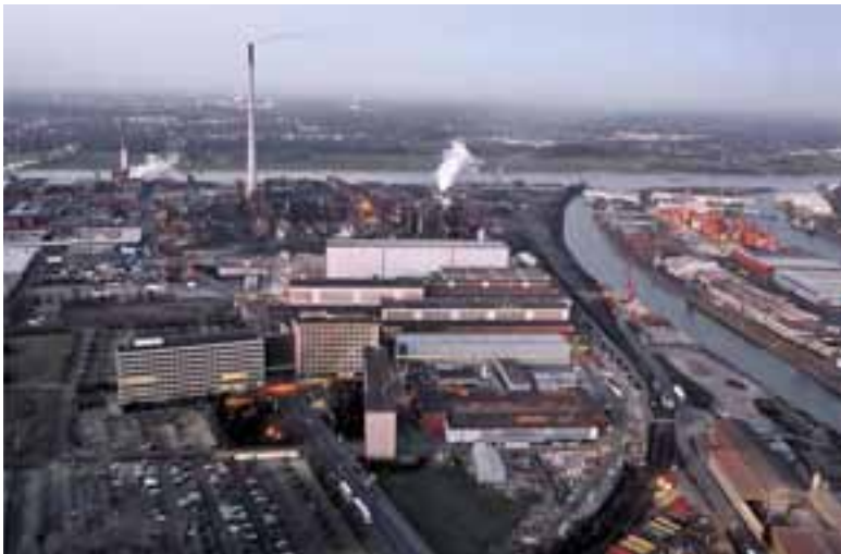
The compressor factory in Duisburg; one of the locations in which the Project Directors Community was able to present its experience and know-how
