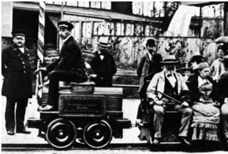
Fig. 1.1: First electric locomotive by W. v. Siemens 1879, Berlin
