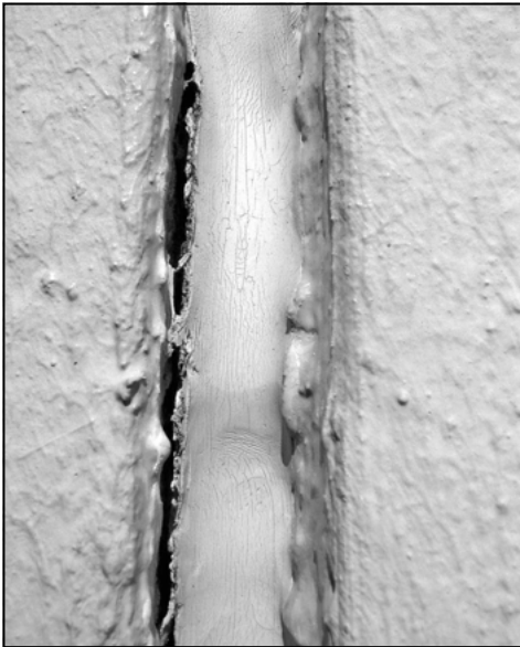
Figure I-2.7: Adhesive failure (left) of a sealant in an expansion joint
