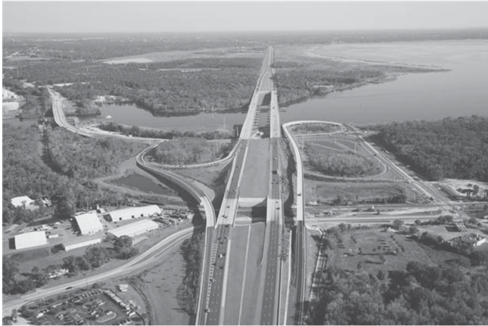
Interstate 4 and 17/92 intersection in Sanford, Florida
