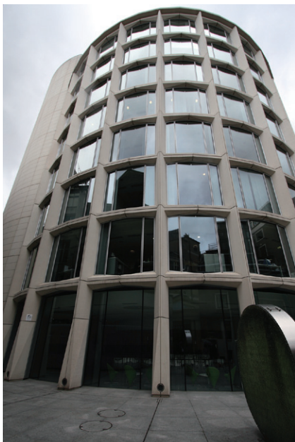
Figure 1.10 Asticus Building, London, 2010. Precast cruciforms form (a) the exterior structure, and (b) architectural finish.
