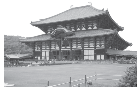
752 AD: Todaiji, Nara. Buddhist temple is world's largest wooden building; present reconstruction is two-thirds of the original temple's size.
