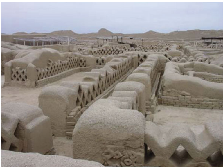
Fig. 1.13 Ruins of a palace constructed in rammed earth technique, built in Chan Chan in present-day Peru in the thirteenth century AD [8]
