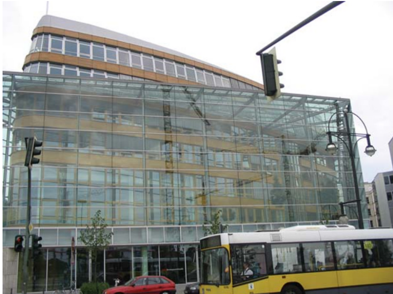
Fig. 1.4 A conventional building enclosed in a glazed outer structure. The two structures appear to be completely independent of each other.
