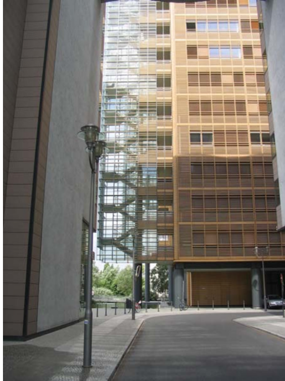
Fig. 1.3 A very visible staircase. How is it supported? You'll learn more about cantilevers later in the book.
