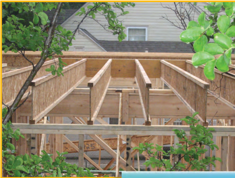
I-joists are engineered lumber products that provide consistency and fewer floor squeaks.
