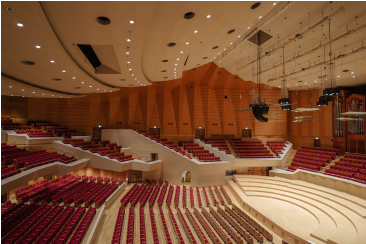
View from side terrace. The ceiling is composed of overlapping plates of gypsum which meet at their highest point just in front of the stage edge. This point is much higher than the elevation of the suspended, plexiglass ensemble reflectors
