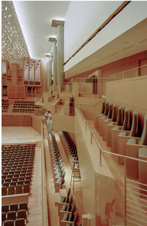
Balcony loges. The blocks of balcony seats are broken into groups and angled towards the stage. This improves sightlines and provides visual interest to the otherwise rectangular plan
