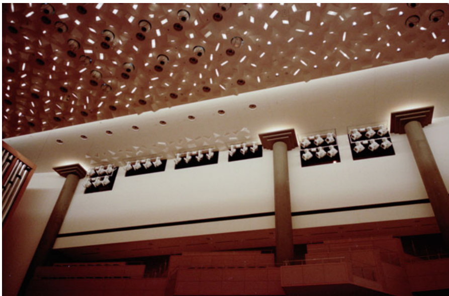
Retractable lighting rigs. At the corner of the walls and ceiling, retractable lighting can be used for specialized performances. When not in use, the white walls are left clean. Spherical lights embedded in the central ceiling panel are used for everyday performances
